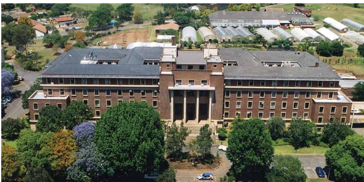
Aerial view of Agriculture Building, Pietermaritzburg.
